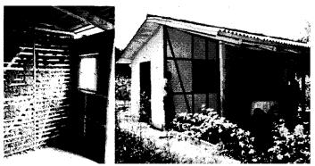
Figure 5. Rural self-help housing developed with a combination of the traditional "torchi" and "quincha" wood and adobe methods developed by the Centro de Estudios Tecnicos NGO.
