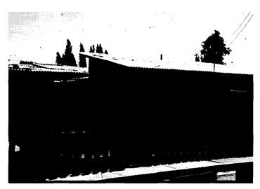
Figure 1. A typical view of a "Caseta Sanitaria" site and service low-income housing. The lots in the first phase include a 100 sq. mt. lot with a sanitary unit of 6.75 square meters. Shown in the picture are two sanitary units together divided by a wood fence and surrounded by the first spontaneous wood housing structures.
